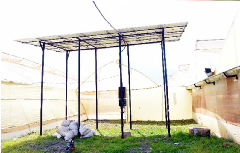
Solar energy in smart greenhouse powers movement motors and sensors
